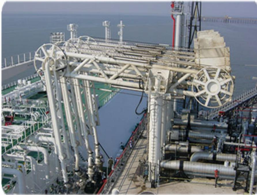
LNG Unloading Arm Installation Example
